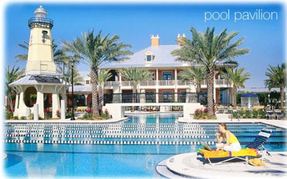
Pool Pavilion Mirabay Development Harbor Bay CDD
